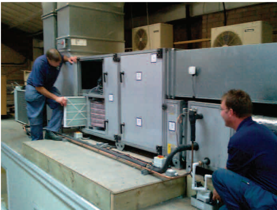
Photo is of the Air Handling Unit installed at Fans & Spares head office which provides Heat Recovery, LPHW Heating & DX Cooling to the sales offices
